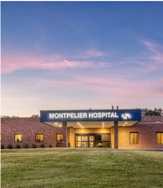
Left: Existing and future institutional buildings, sites, and campuses within a community offer key services for residents and improve quality of life.
