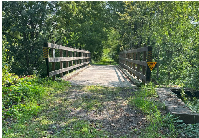
Photo 6 Bridge over Beaver Creek
