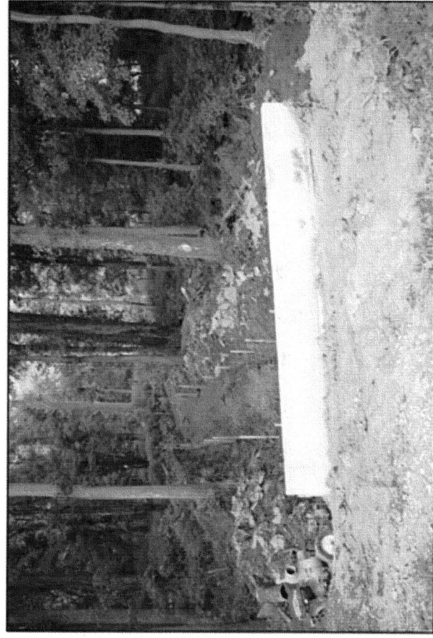
PHOTO BY JENNA FRISBY, THE VILLAGE REPORTER The Iron Horse River Trail Senior Center Trailhead is currently closed while the trail undergoes the construction of making the trail into an asphalt pathway which would include two bike lanes as well.
