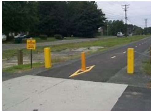
Photo 10 Bollards at Access Points
