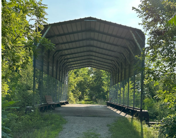
Photo 5 Bridge over County Road 15
