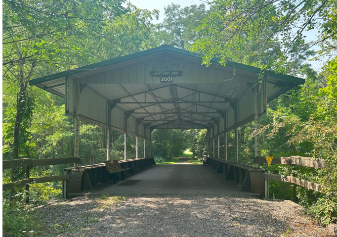
Photo 7 Bridge over County Road 20-40 (Liberty Street)
