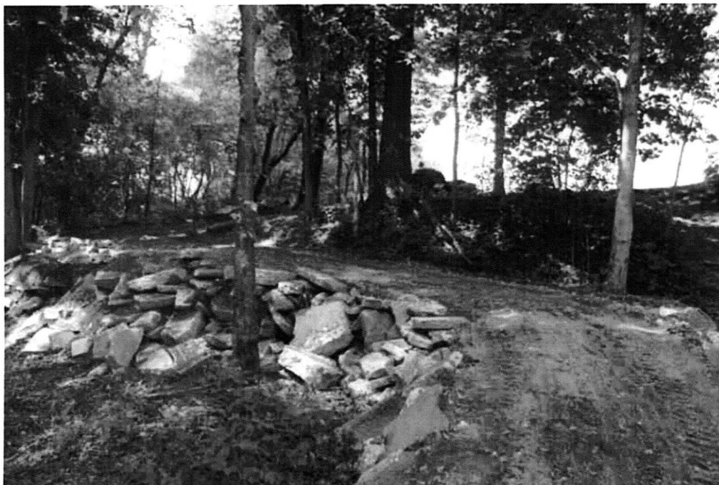
TRAIL WORK ... The St. Joe River Trail where work was done to elevate part of the trail so that it is safer and not as steep of a drop when walking or biking.
